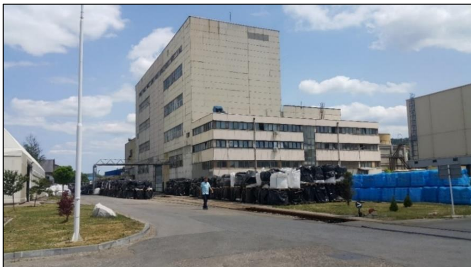
Figure 10. Vacuum evaporation plant within the Solana Saltworks (photograph taken by Tijana Veljković in June 2022)
